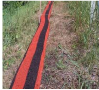
Compost Filter Sock
