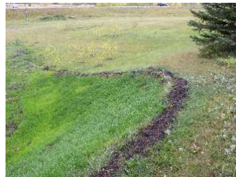
Blanket Installation and Result
