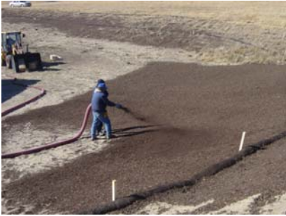
Compost Blanket installation
