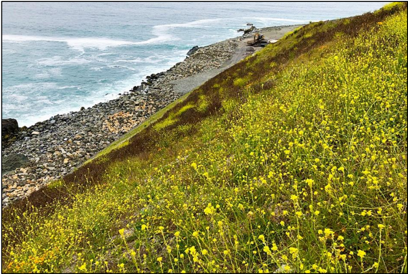
Coastal application of composted mulch. Photo courtesy Z-Best/GreenWaste
