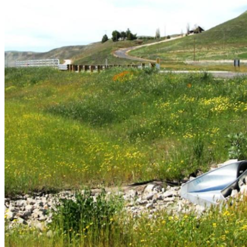
Education of specifiers about compost usage, such as in bioswales (above), is key to seeing continued growth in highway and large construction project applications.
